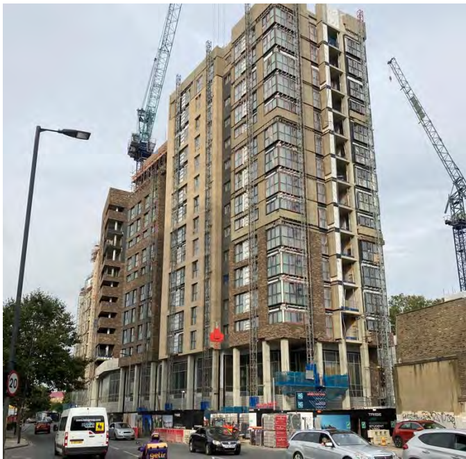
Ilderton Road, view of 313 Student Housing scheme
