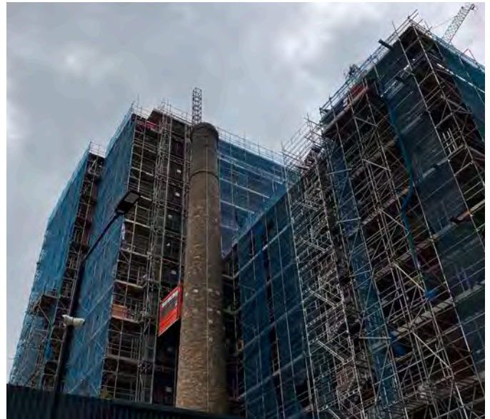
Glengall Road Chimney
