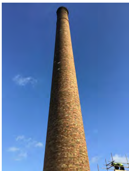
Glengall Road Chimney
